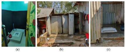
Figure 7: (a) Showing Permanent Built Attached Toilet with Fine Finished Material in Good Condition and (b), (c) Very Poor Temporary Built Common Toilets and Bath Facilities.
